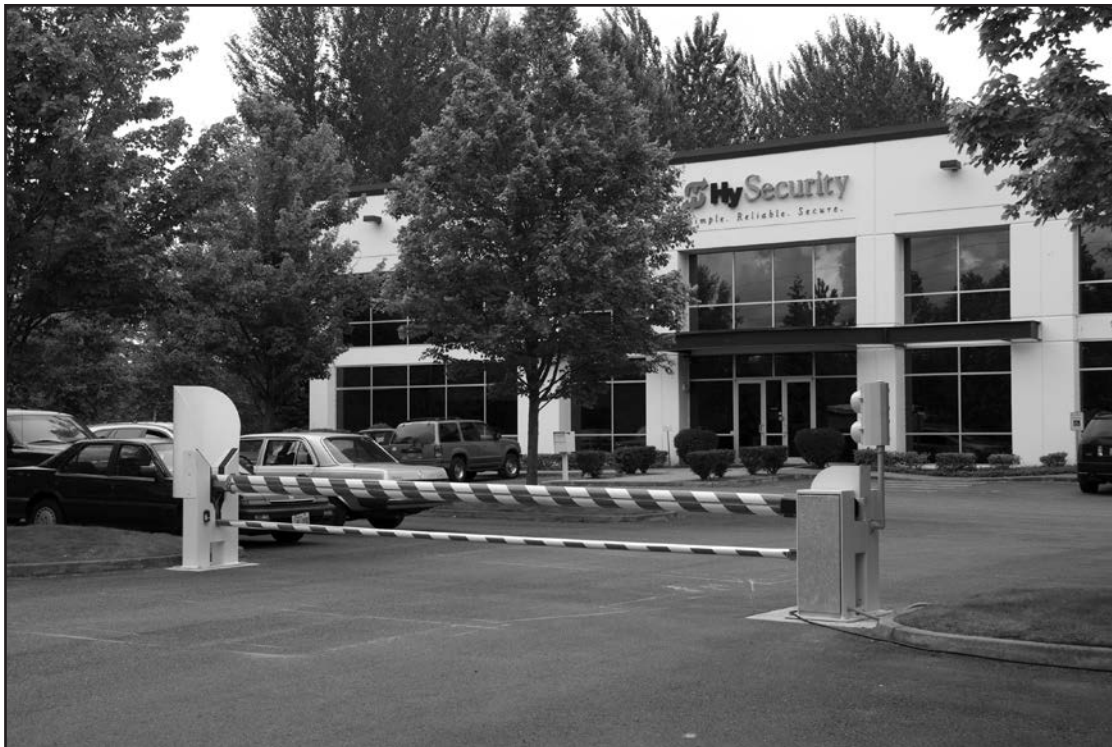
HySecurity Gate, Inc. Headquarters in Kent, WA
