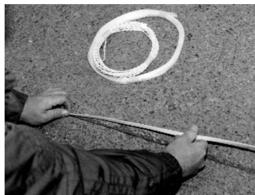
Saw Cut Loop
