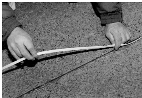
Saw Cut Loop
