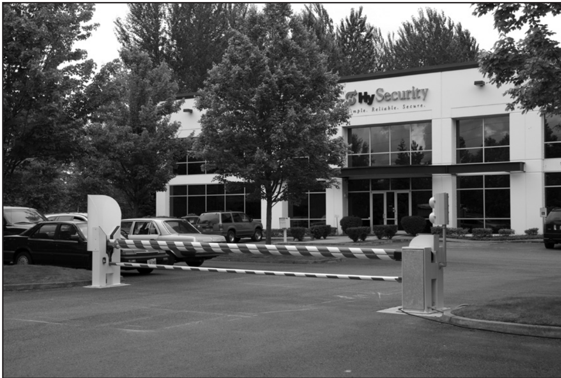
HySecurity Gate, Inc. Headquarters in Kent, WA
