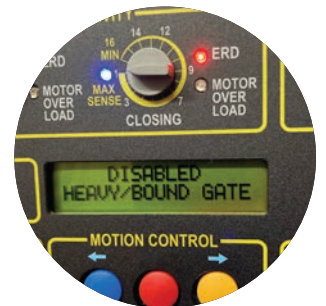
Heavy gate or binding gate detected
