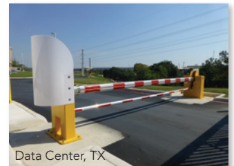
Data Center, TX
